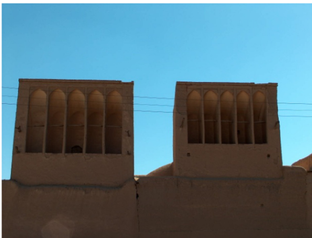
Fig. 13. A view of a one-sided wind tower in Ardakan city, Yazd province, Iran [1].
