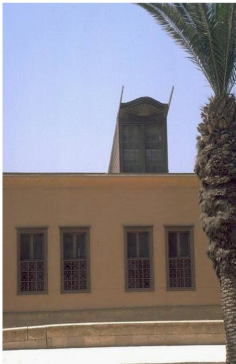
Fig. 2. The one-sided wind tower of a house in Al-Jawhara in Cairo, Egypt [12].
