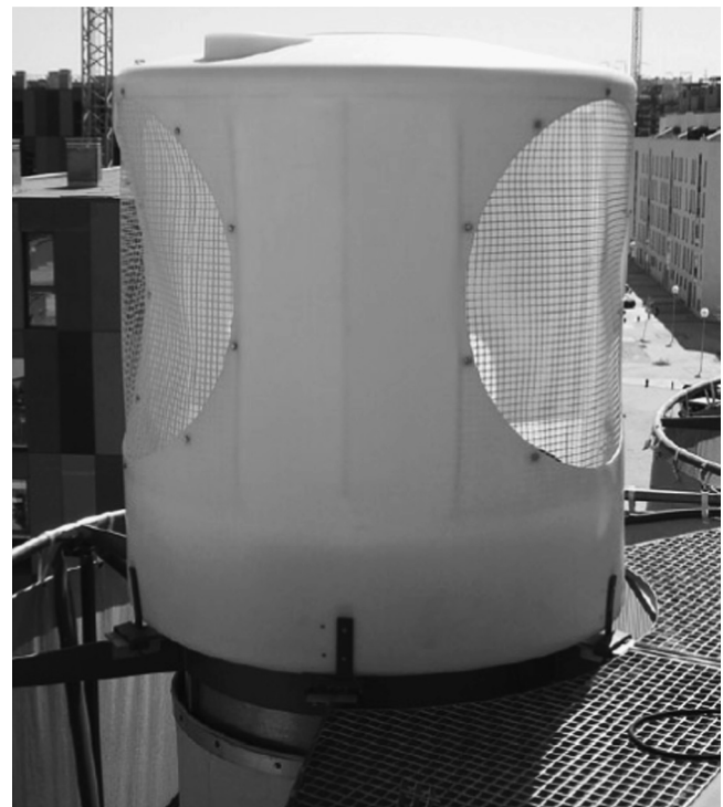
Fig. 9. View of the wind catcher installed at the top of each tower shown in fig. 8 [37].
