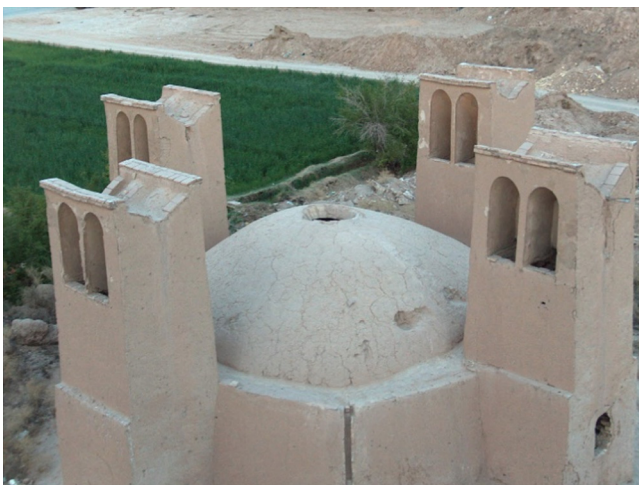
Fig. 14. Two-sided wind towers of the underground water reservoir in Dowlat Abad Garden, Yazd, Iran [1].
