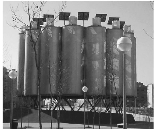
Fig. 8. View of the cylindrical evaporative wind towers in Madrid [37].
