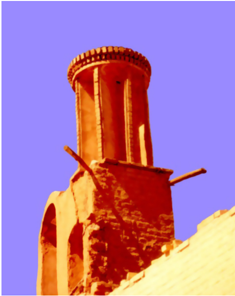
Fig. 16. A cylindrical wind tower in Yazd, Iran [1].
